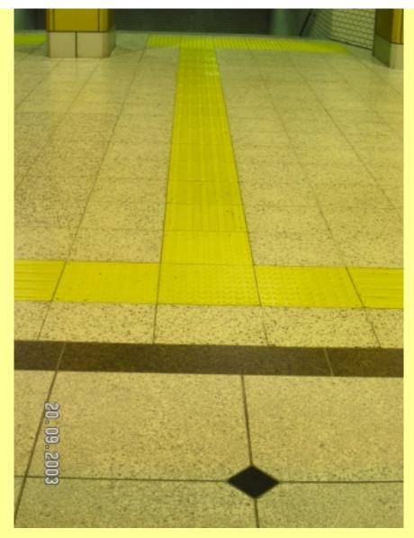
THE ABOVE YELLOW PATHWAY WHICH HAS A ROUGH CONTOUR PERMITS A BLIND PERSON TO FIND HIS PATH USING A BLIND STICK. THIS PICTURE IS FROM A RAILWAY STATION IN JAPAN.
